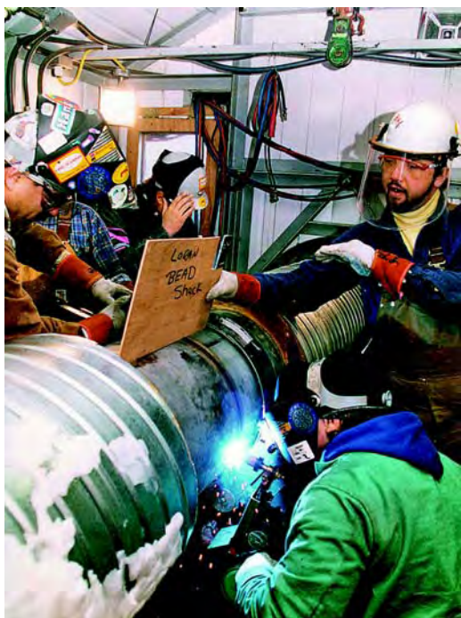
大口径双相不锈钢管道的机械化焊接 (来源: Arco Exploration and Production Technology)
