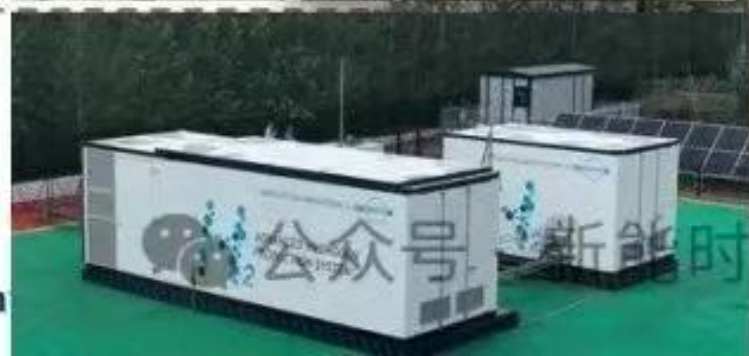
清华碱液制氢设备 Tsinghua Alkaline Hydrogen Production Equipmen
